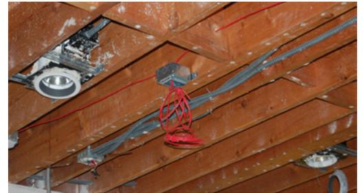
*The red wire electrical box is for the smoke detector system. Notice the hole in the blocking through which the red wire passes which needs to be sealed.*
