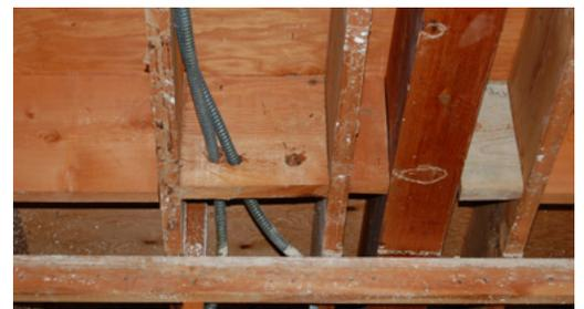
*Electrical flex conduit needs fire caulking (red color) and the drilled hole in the blocking needs to be filled in.*
